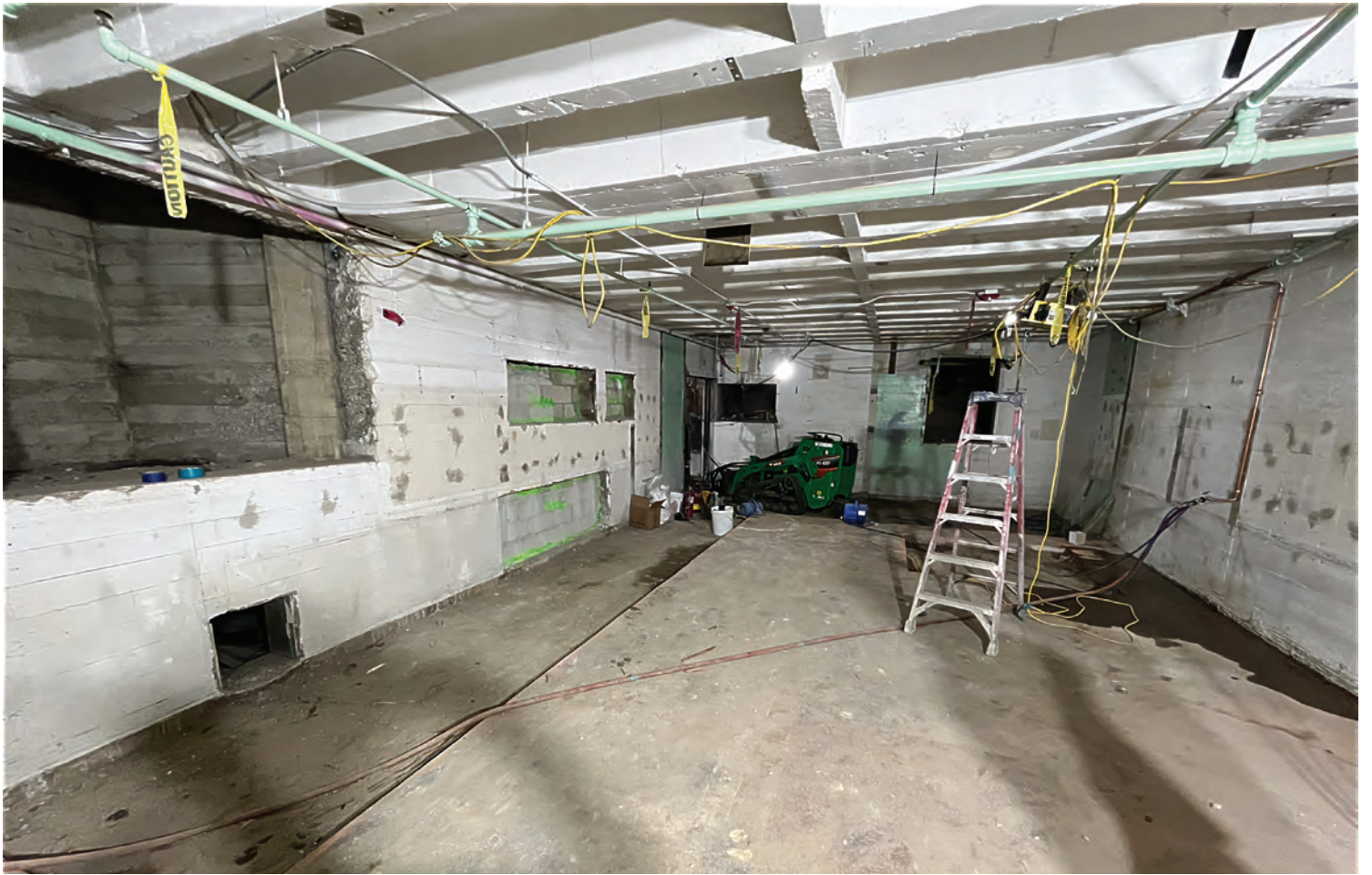
Primary Dressing Room current state January 2025
