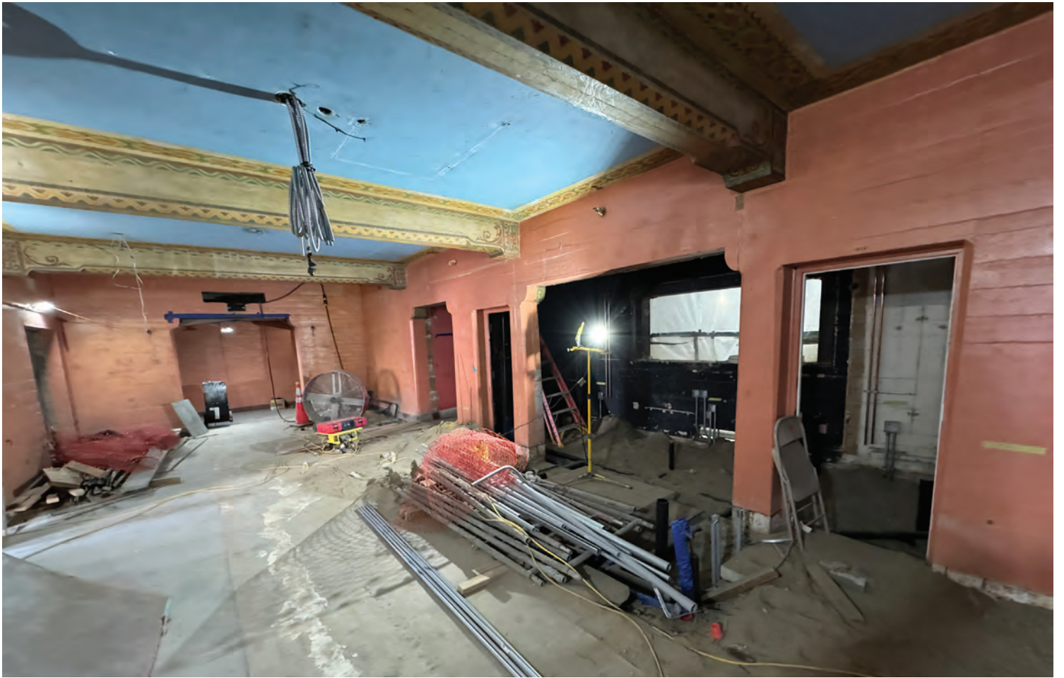
Lobby as of January 2025
